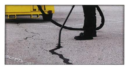
cleaning the cut surfaces and placing the specified materials into the cavity to prevent the intrusion of water and incompressibles into the crack.
