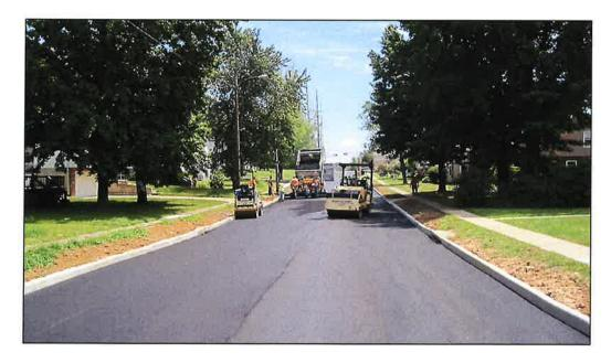
**Existing Pavement Condition:** The existing pavement should exhibit a good base condition. The visible surface distress may include: severe surface raveling, multiple longitudinal and transverse cracking with slight raveling, a small amount of block cracking, patching in fair condition, debonding surface and slight to moderate rutting.
